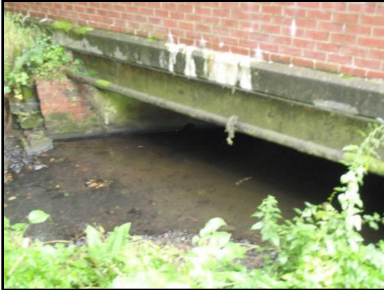
Figure 4 - Road Bridge over Hepscoth Burn
