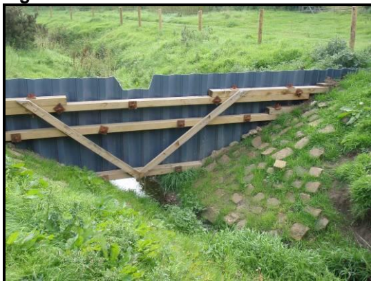
Figure 6 - Tranwell Farm weir structure
