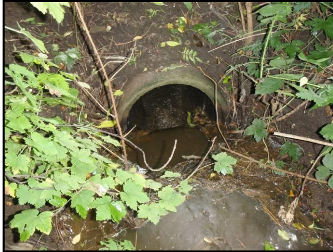
Figure 3 - Crofts Park Culvert entrance
