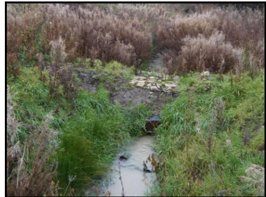
In channel flow control bund down stream of farm access track
