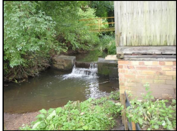
Figure 5 - Weir structure in watercourse
