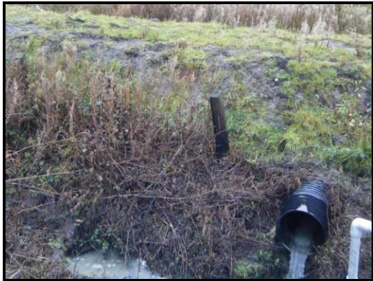
Environment Agency embankment and outfall into Red House Burn
