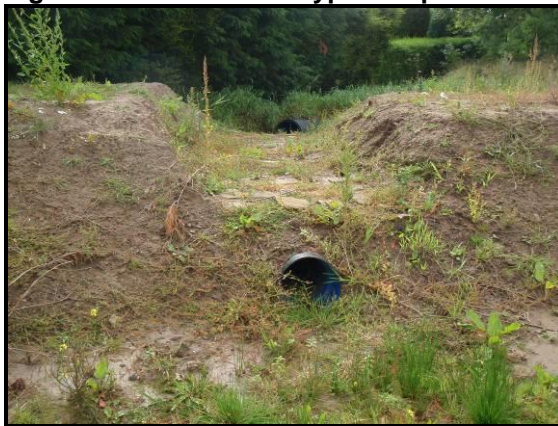
Environment Agency embankment and Outfall
