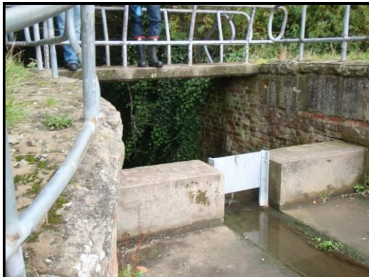
New Environment Agency stop board at pond outfall to increase storage in pond
