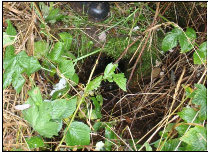
Figure 2 - Orchard Culvert Entrance
