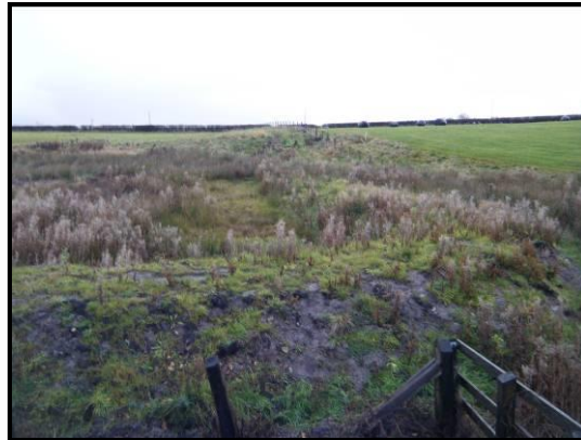
Environment Agency embankment and storage area
