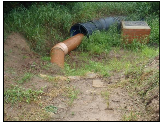
Secondary embankment and connection with larger 600mm bypass pipe
